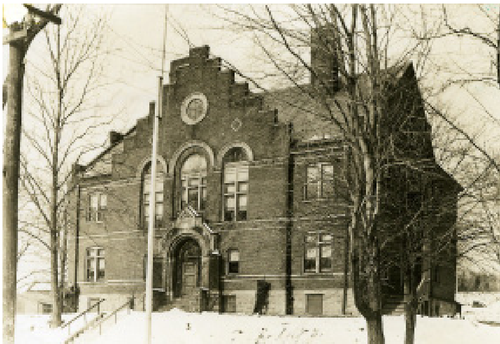
Short Hills Elementary School, Hobart Avenue, Short Hills
