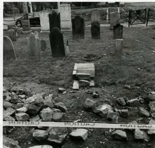
Stone work and wall repair at Parcil Cemetery.
