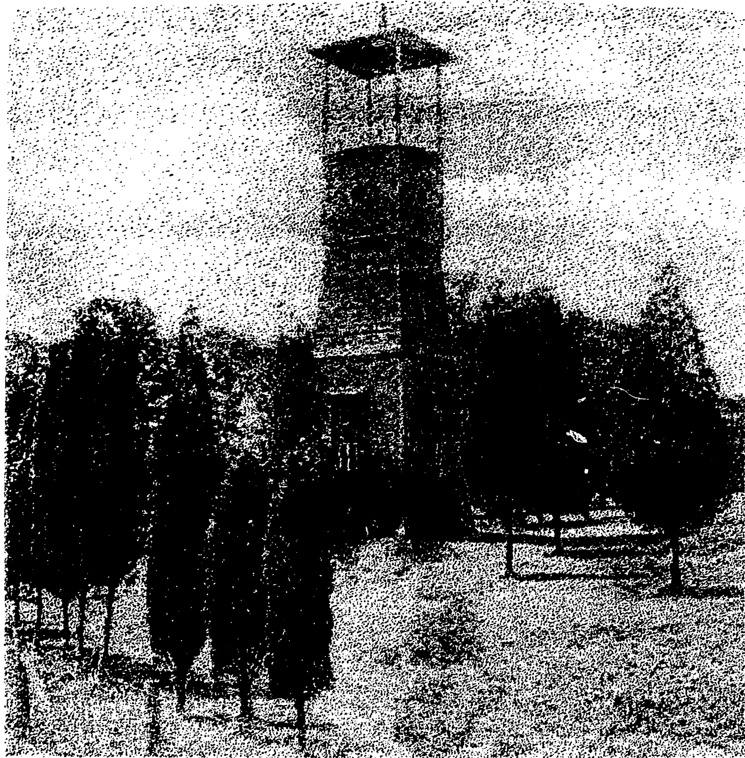
(In the 1947 book The Development of a Community , the photo above is identified as "The Old Tower, once a rotary windmill, which stood on the grounds of the late Stewart Hartshorn, near the Short Hills Station. Its original purpose was aiding in the local water supply.")
